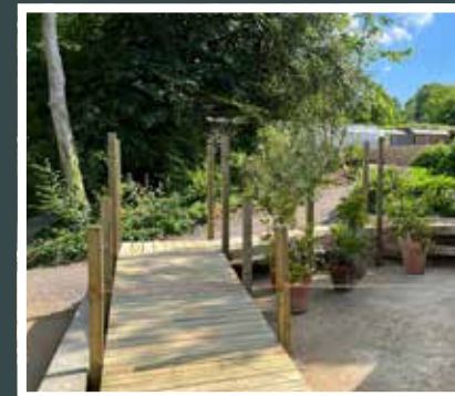
Access ramp under construction
